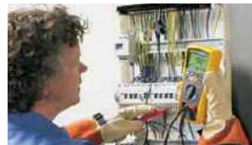
Insulation test at a distribution panel
