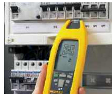
Location of fuses/breakers and assignment to circuits
